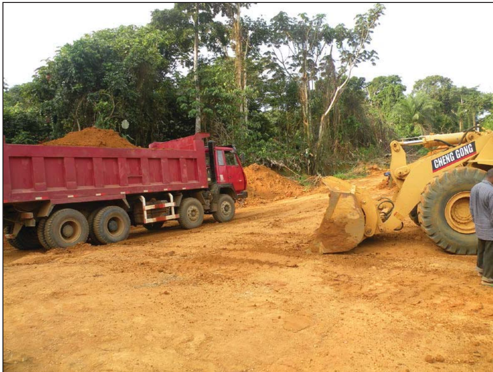
Photo 2 - "Route nationale 3" Kisangani–Bukavu (DRC): rehabilitation works
